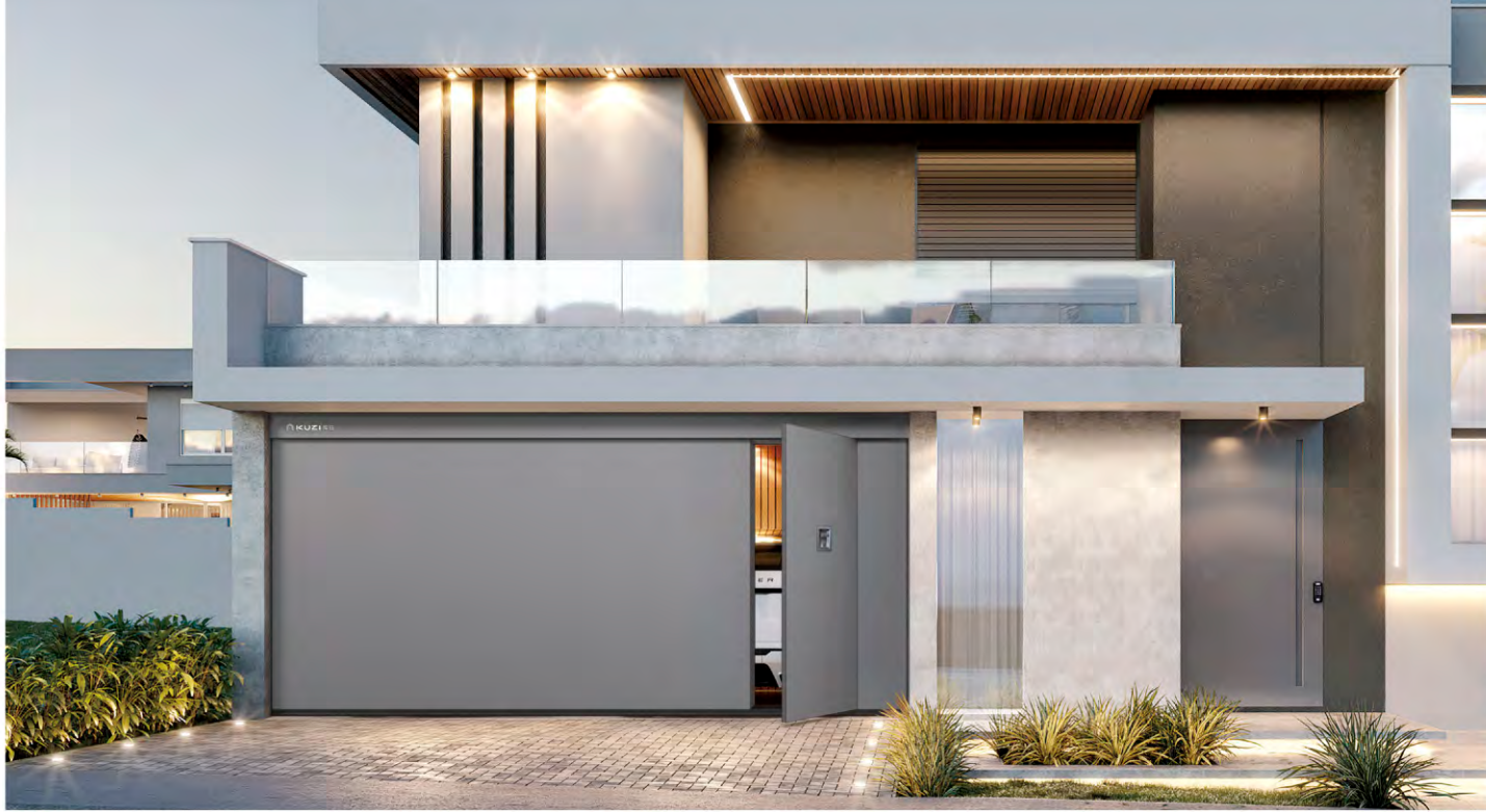
SAFETY DOOR INTEGRATION SYSTEM OF VILLA GARAGE
